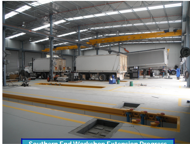
Southern End Workshop Extension Progress
