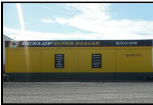
Dunlop Super Dealer shed located at Tatiara Truck & Trailers
